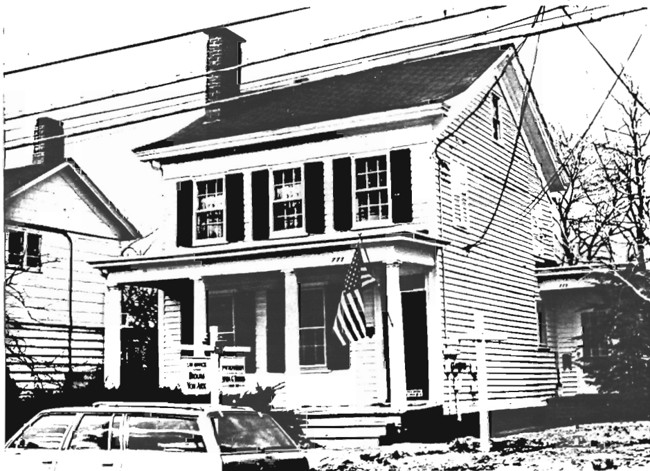
1313-1-14. 777 River Road. Block 49, Lot 2. Neg. File No. 2-19,20,28. Greek Revival house, c.1850-1860. 2½ story 3 bay by 2 bay rectangular side-hall plan, with 1 story rear ell. Gable roof with slightly flared eaves and box cornice; 2 interior end chimneys; brick foundation; clap- board siding. 6/6 sash windows; narrow asymmetrically-placed entry with 2-light transom and 6-panel door. Full porch has octagonal columns. Early mapping not clear; owner possibly C.C. Hendrickson in 1860; J. Chadwick in 1873 and 1878; Mrs. Smith in 1889.
