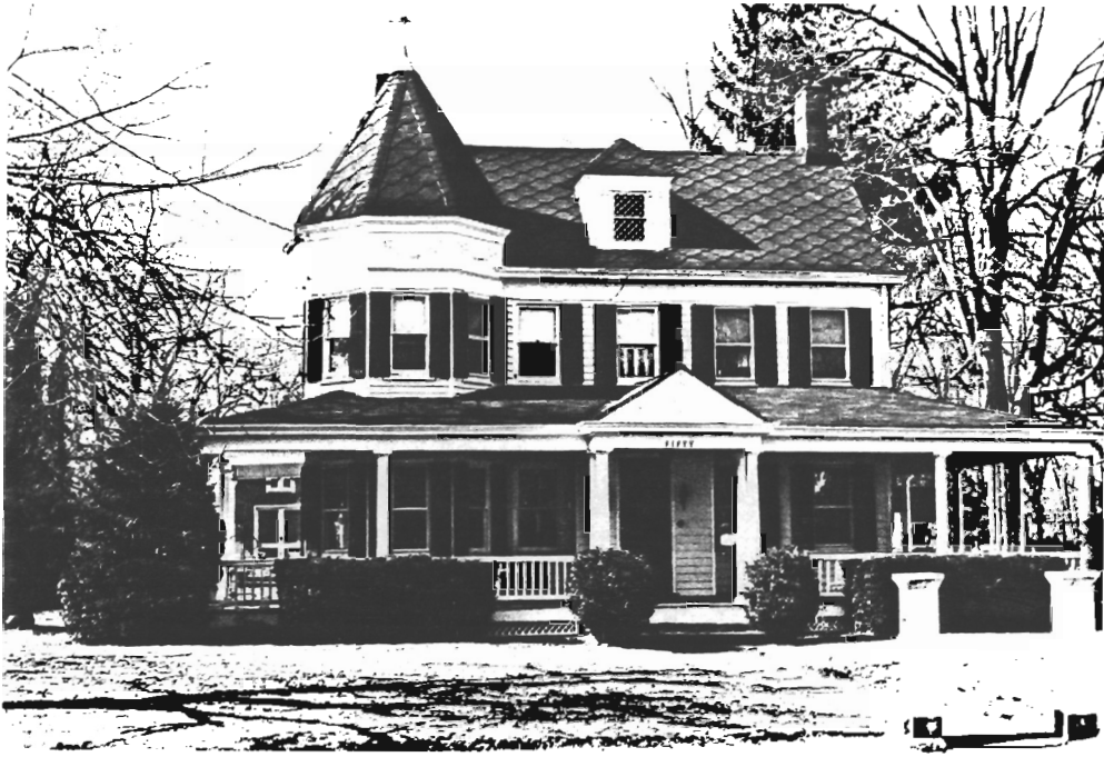
1313-1-6. 50 Fair Haven Road. Block 27, Lot 6. Neg. File No. 1-30,31,32,33. Queen Anne style house, c. 1890. 2½ story complex plan with a broad veranda on 3 sides and a polygonal turret. Gable roof; 2 interior end chimneys; clapboard siding; scalloped shingles on gable ends and dormer. Wide frieze with swags in relief; pilastered dormer with small diamond lights; 1/1 sash windows; paneled door with upper glass light; Doric columns and pedimented gable on veranda. Well conserved.
