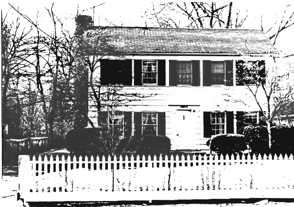
1313-1-4. 40 Fair Haven Road. Block 27, Lot 8. Neg. File No. 1-26. 5 bay I-house, c. 1850-1870, with later alterations. 2 stories; gable roof; exterior end chimney; wood shingle siding (2nd story of main facade has vertical boards). 6/6 sash windows with louvered shutters; 6-panel door with slender pilasters and wide entablature. 1907 map shows front porch on north end. Early mapping is ambiguous; S. Hendrickson owns house on 1873, 1878, and 1889 maps.
