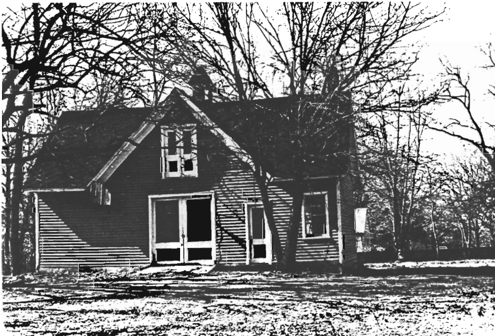
Carriage house and stable, rear of house. Rectangular plan with cross gable roof, clapboard siding, diagonal-panel doors, and a small cupola.
