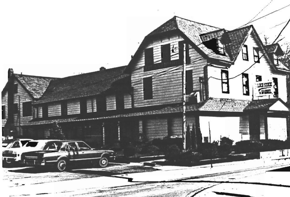
1313-1-13. 121 Fair Haven Road. Block 52, Lot 26. Neg. File No. 1-9,10. Atlantic Hotel, c. 1885. Now Lock Stock n Barrel Restaurant. Founded by Stout Holmes Bennett, this wood-frame hotel is 2½ stories, 4 bays by 2 bays, with long 2 story rear ell addition. Front section has jerkinhead roof with slate tiles. Interior and exterior chimneys on ell. Shingle siding. Concrete veneer (over brick?) foundation. 2/2 sash windows. Poor 1st story alteration. Building originally had clapboard siding, lou- vered shutters, and porch on 3 sides with Stick Style trim.
