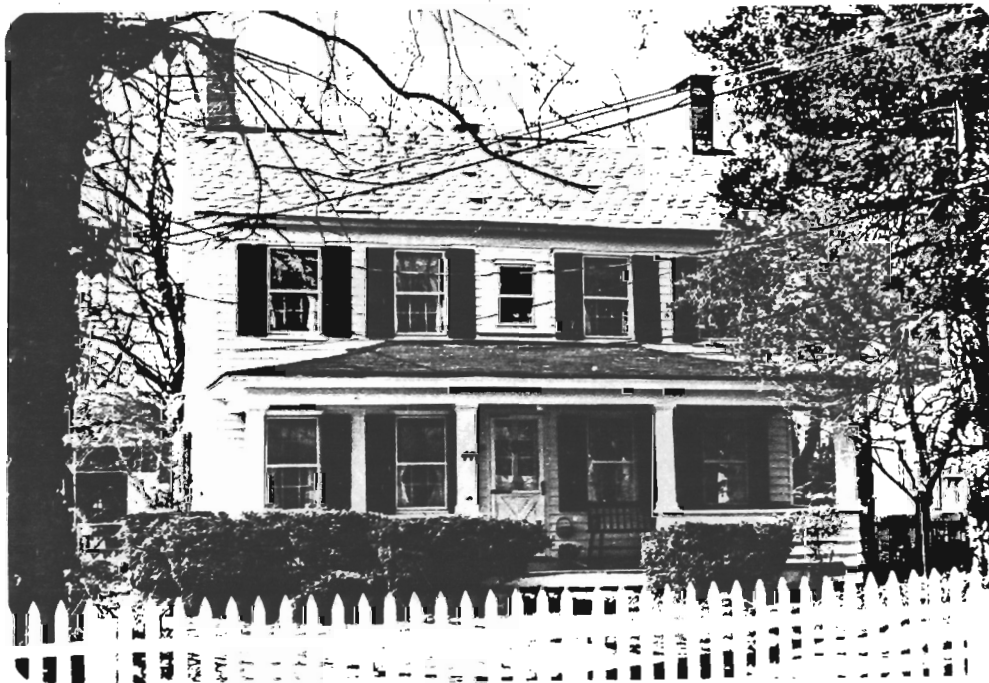
1313-1-5. 44 Fair Haven Road. Block 27, Lot 7. Neg. File No. 1-27, 28, 29. 5 bay I-house, c. 1850-1870, with later alterations. 2 stories; 1 story rear ell; slate tile gable roof; 2 interior end chimneys and 1 internal chimney; clapboard siding. 6/6 sash windows; simple doorway; full porch with square posts dates from early 20th century. Early mapping is ambiguous; William B. Little may be original owner. Mrs. Little is owner on 1873, 1878, and 1889 maps.
